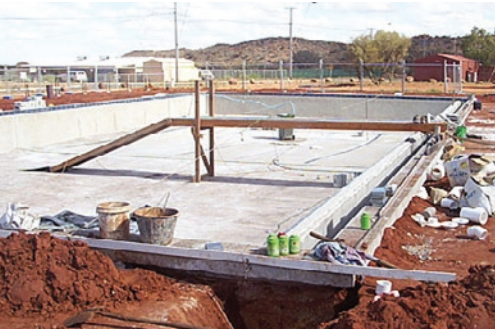
Pool layout & excavation established. Concrete floor poured.
