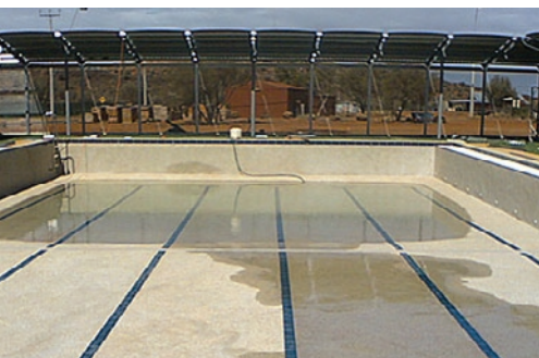
Pebble finish & six lane tiles completed.
