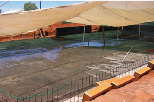
Pool is fully concreted. Blue Gloss water line tiles applied.
