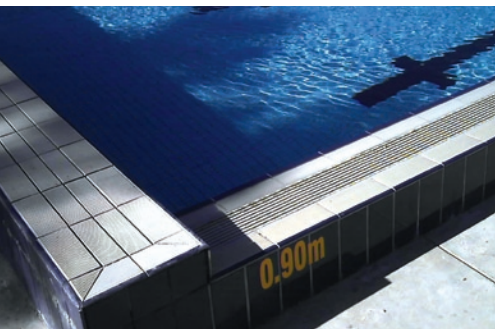
Image of renovated scum gutter to wet deck
